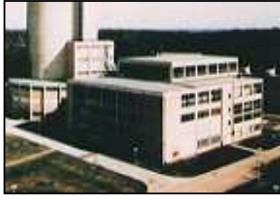
AVR, Germany 15 MWe 1967-88
