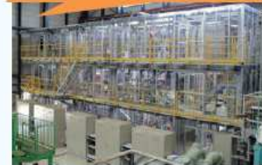
H 2 production test facility
