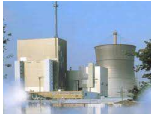
THTR, Germany 300 MWe 1986-89
